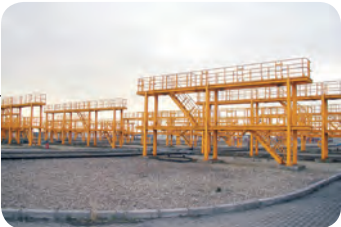
リーファ電源 Power points for a refrigerated container
